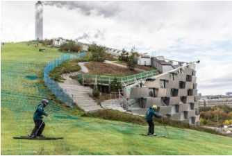
Copenhill Amager Bakke, Copenhagen, Danimarca © SLA
